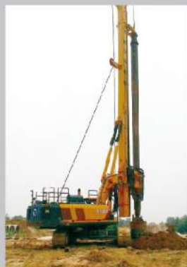
陇海路高架延伸栎阳段，施工快速高效 XCMG rotary drilling rigs were working in express way with high efficiency
