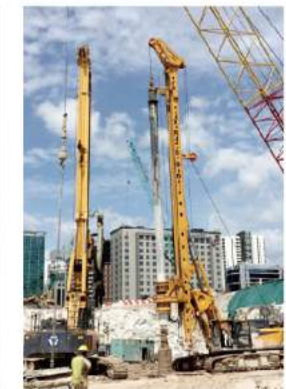
XR280DII马来西亚吉隆坡施工 XR280DII working in Kuala Lumpur, Malaysia
