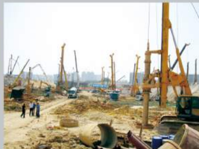
徐工旋挖钻机在南宁火车站施工 XCMG rotary drilling rigs are working in Nanning Train Station
