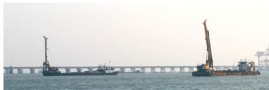
徐工旋挖钻海上展雄风 首次实现多台钻机海底成槽作业 XCMG rotary drilling rigs are making trench on the seabed
