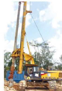
XR220D新加坡施工 XR220D working in Singapore
